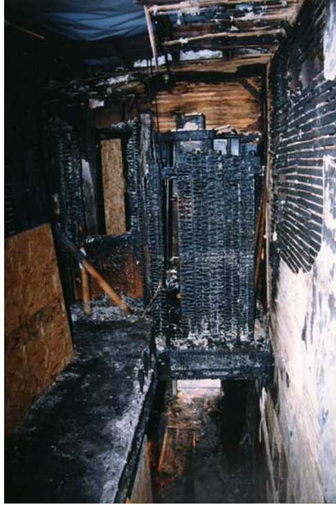
Figure 11. Second floor landing and stairwell looking toward front of structure.
