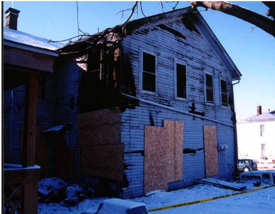
Figure 2. Back of structure.
