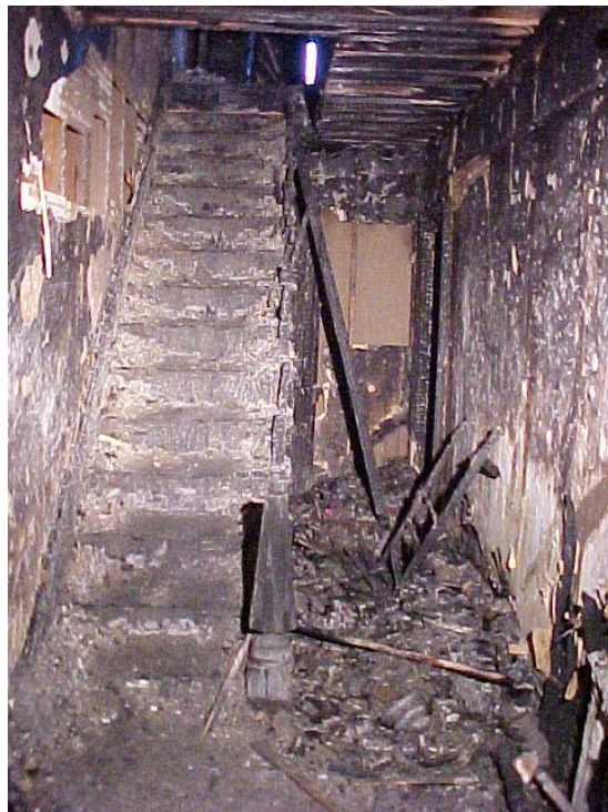
Figure 10. Stairway and 1 st floor hall from front doorway.
